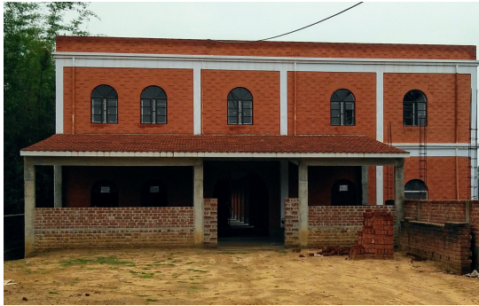
All the walls were rendered with lime and brick dust, the outside waiting freshly built.
